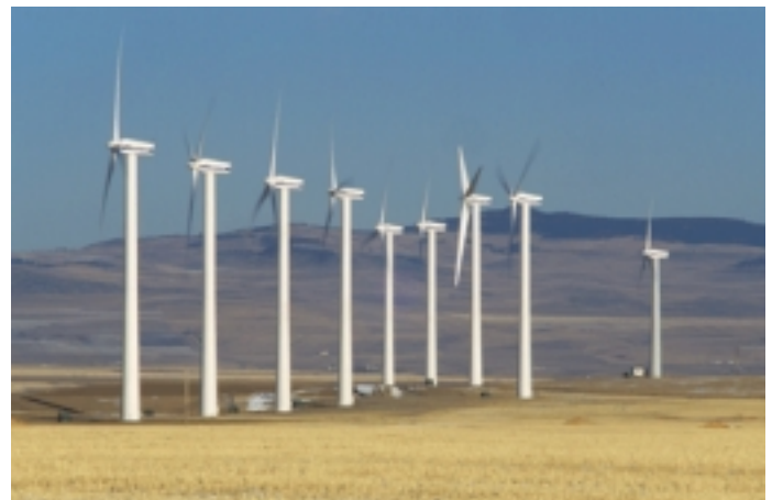
The wind farm at Castle River, Alberta, generates enough electricity to meet the needs of several thousand Canadian homes.
