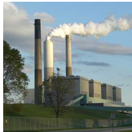
WAR ON COAL: Ontario will shut down all of its coal-fired power plants. Pictured: Lambton generating station in Ontario. Image: Flickr/Toban B.
