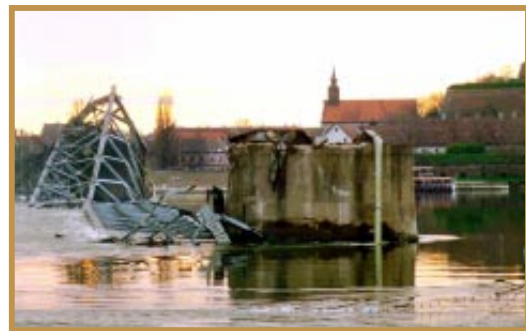
WATER SUPPLY LINE in Novi Sad, Yugoslavia, was destroyed along with this Danube River bridge during a NATO airstrike in April 1999.
