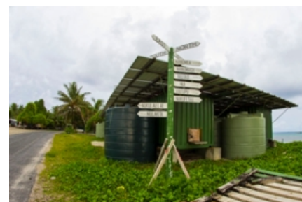
Solar desalination plant on the island of Funafuti in the Tuvalu islands.
